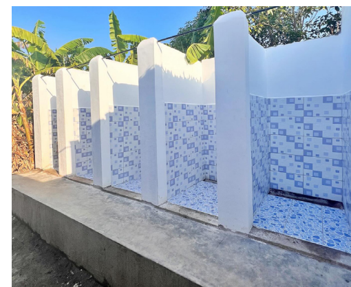
Newly constructed shower facilities.
