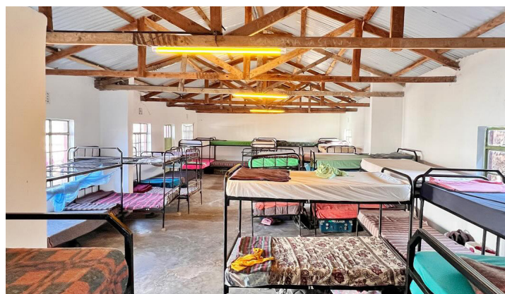
Recently renovated dormitory to comply with new government regulations.
